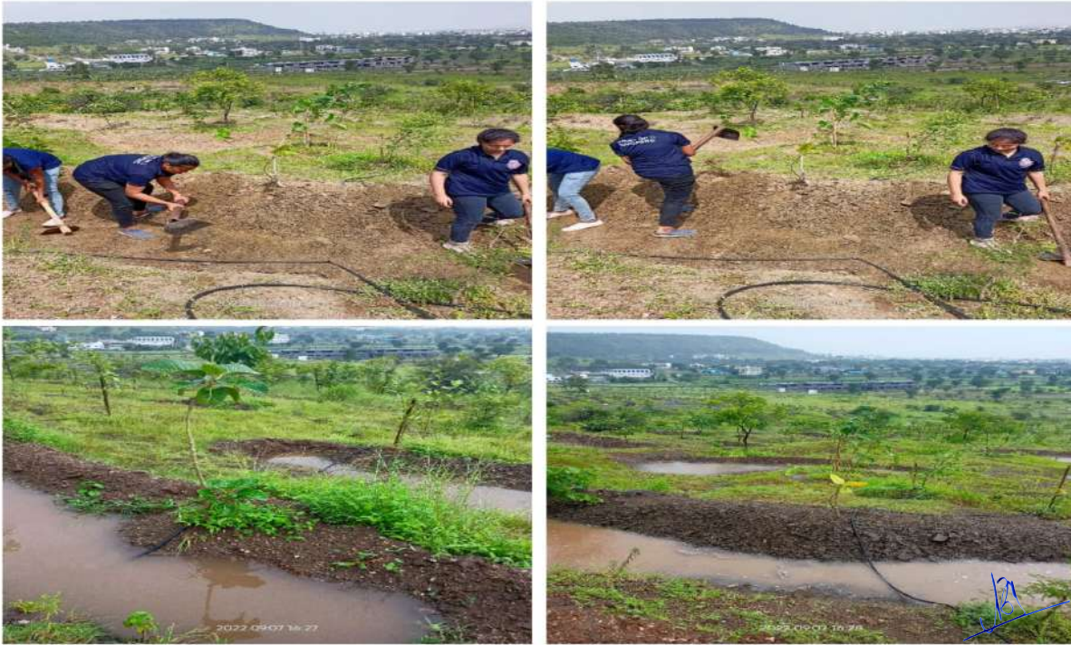
Impact of work done for the purpose of water conservation by digging continuous counter trenches(CCT) on the Bakori hills.
