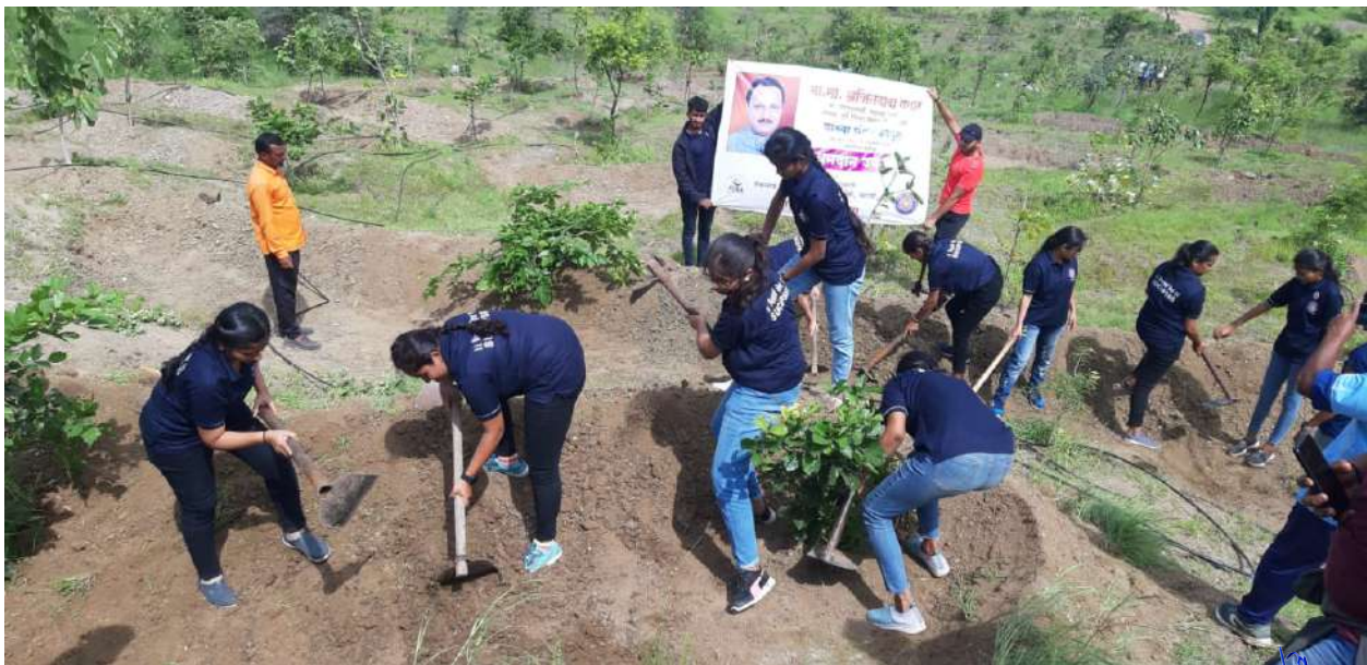
Work for the purpose of water conservation and water horizontally by digging continuous counter trenches(CCT) on the Bakori hills. PRINCIPAL Pune District Education Association's Shankarrao Ursal College of Pharmaceutical Sciences & Research Centre, Khoradi, Pune-411014.
